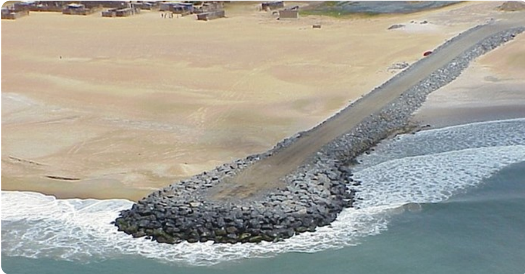
Groynes at the Keta Sea Defense Project on Ghana's coast. Kwasi Addo Appeaning
