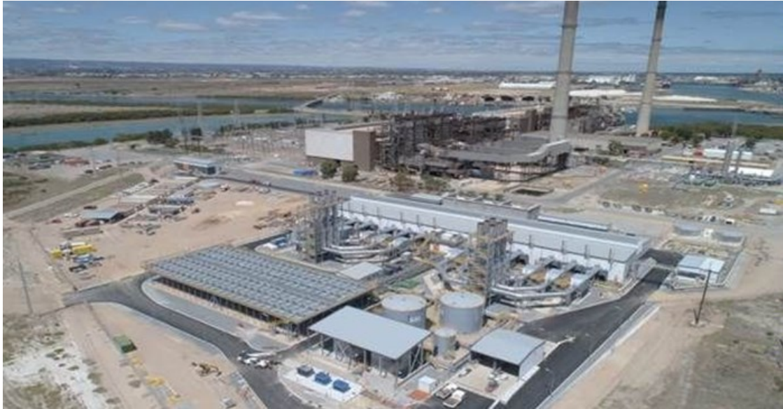
AGL Energy Limited undertook a successful transformation of an old coal plant to a modern flexible gas engine power plant to support more renewables into the South Australian power system
